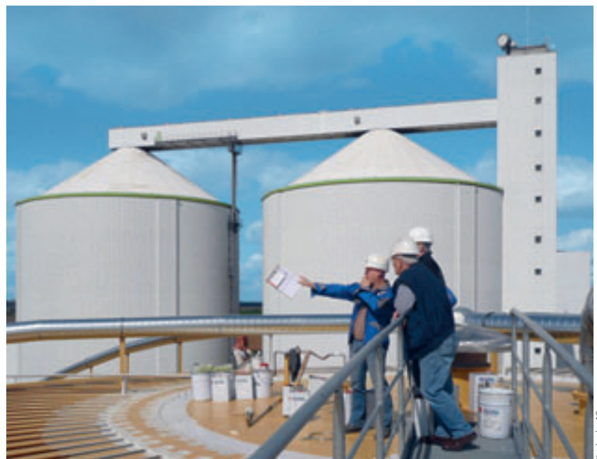
Additional thick juice tanks increased production capacity for Nordzucker
